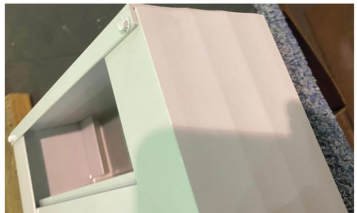
Double Catch Gutter Top Overlap Detail
