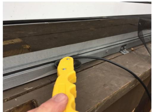
**Inserting Spline for Screen**
